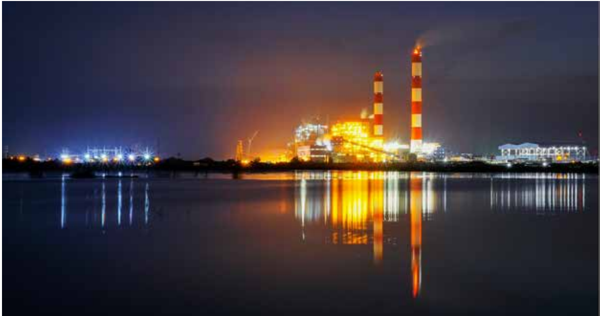
Duyen Hai Thermal Power Plant
