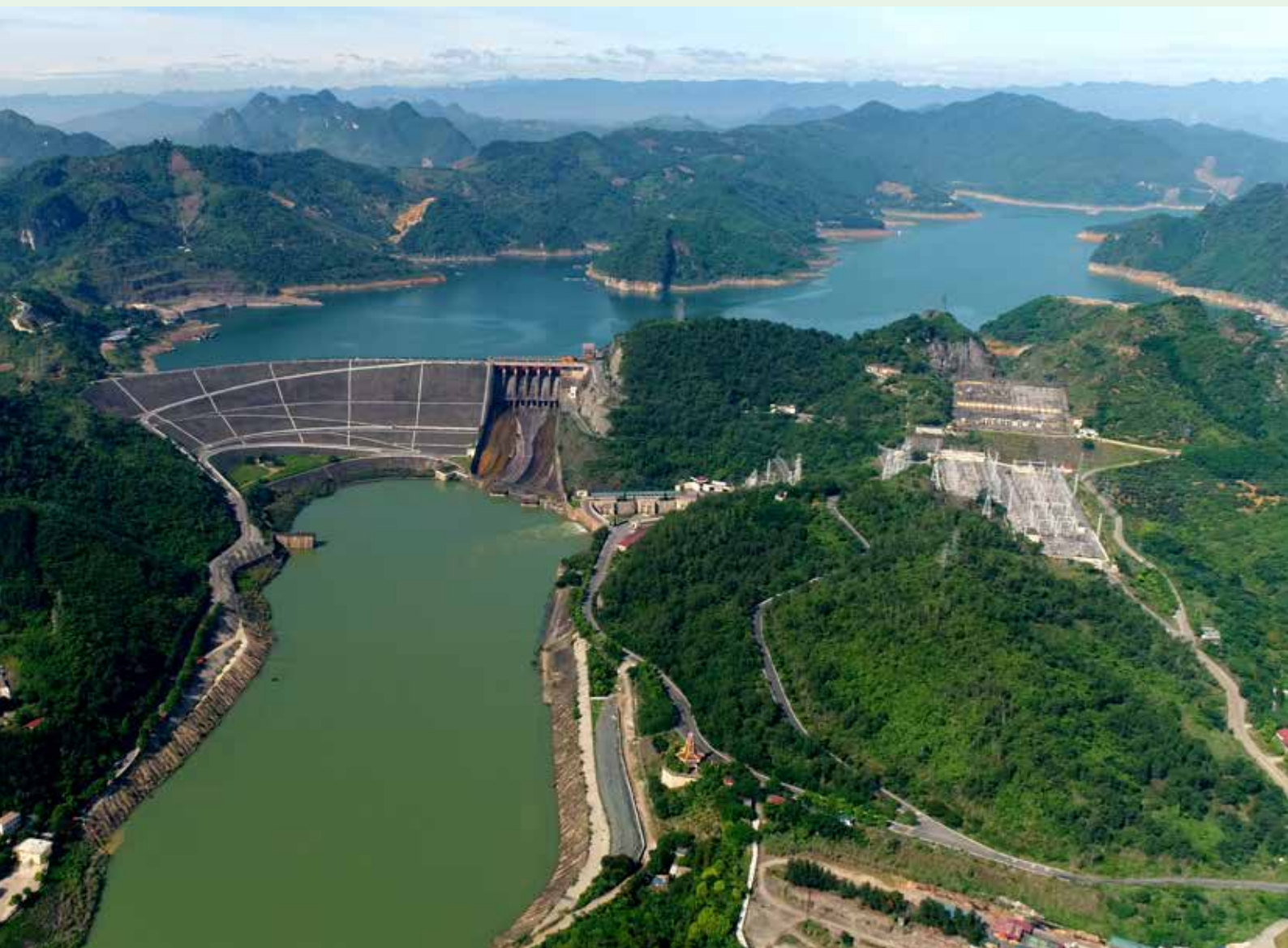
Hoa Binh Hydropower Plant
