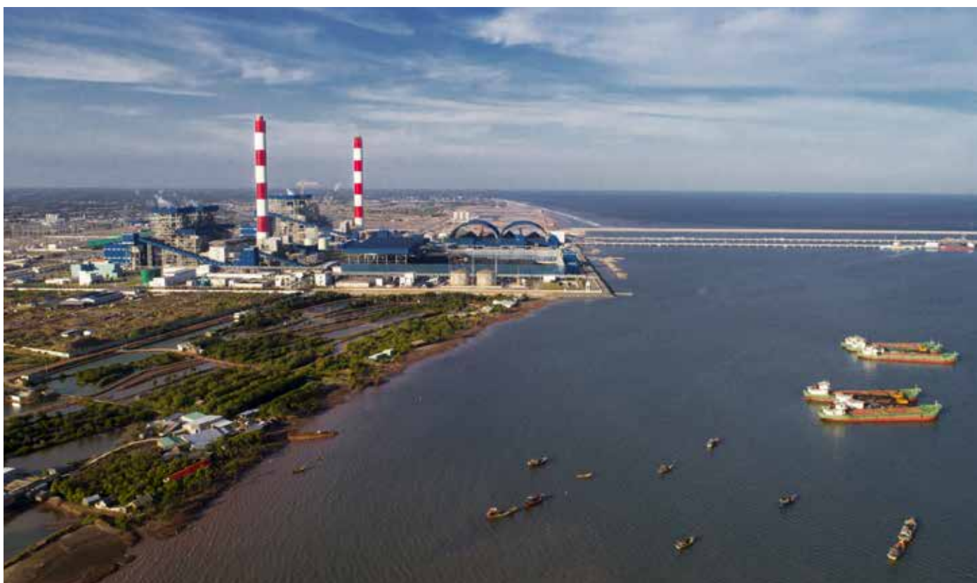
Duyen Hai Thermal Power Plant
