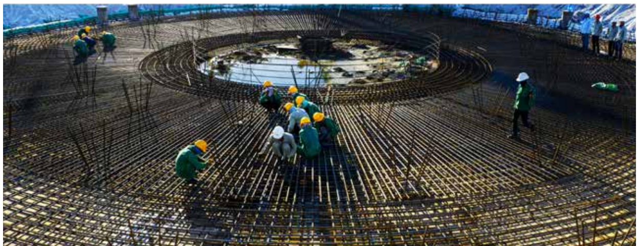
Duyen Hai 3 Thermal Power Project
